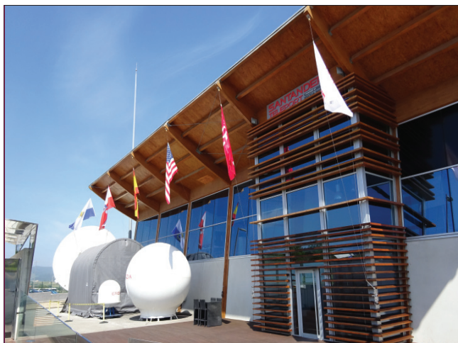
Santander Teleport Main Offices ● ● ●
