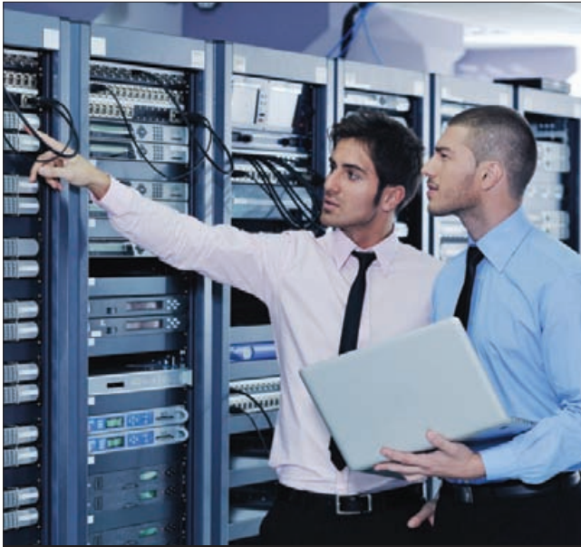
Marlink NW Server Room. Photo courtesy Marlink ●●●
